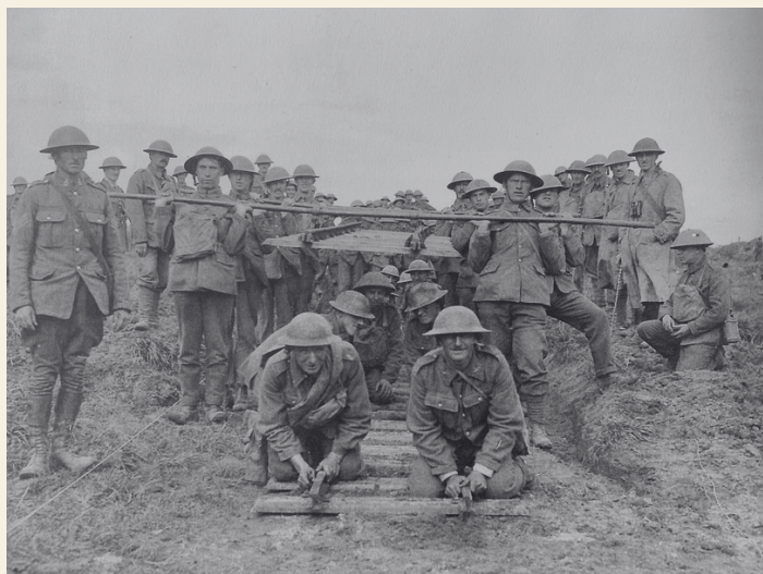
Figure 1: Canadian Railway Troops laying narrow gauge track (Imperial War Museum Q35499)
