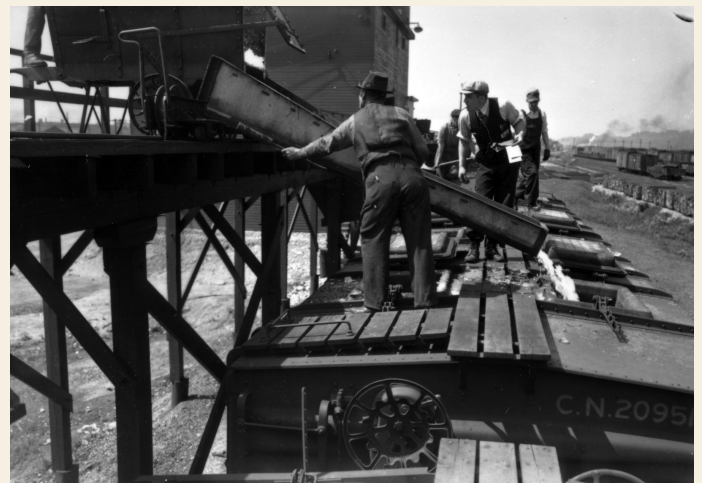
(Icing refrigerator cars at Canadian National's Pointe-Saint-Charles, Montreal, 1941. Photo Courtesy Canadian Museum of Science and Innovation)
